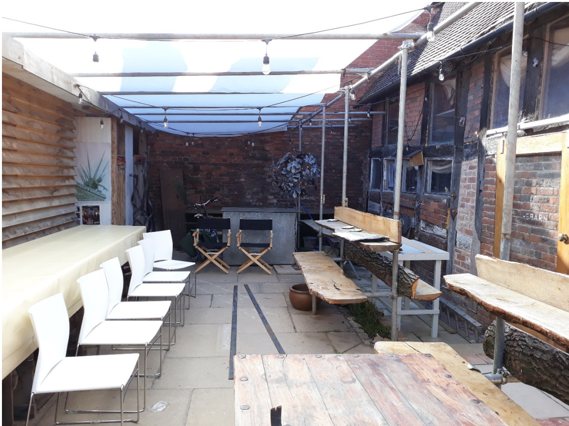
St Katherine's Barn – East Elevation
