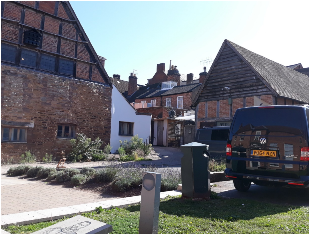
Front of St Katherine's Barn and Alms Houses
